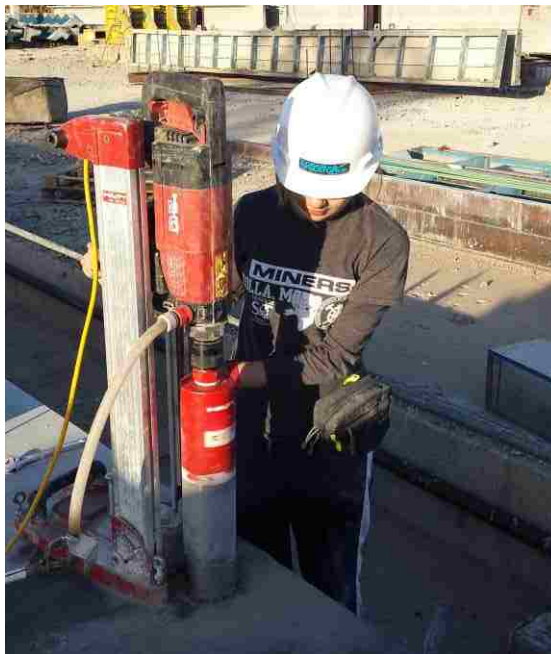
Figure 5.18 Extracting cores from a beam.
