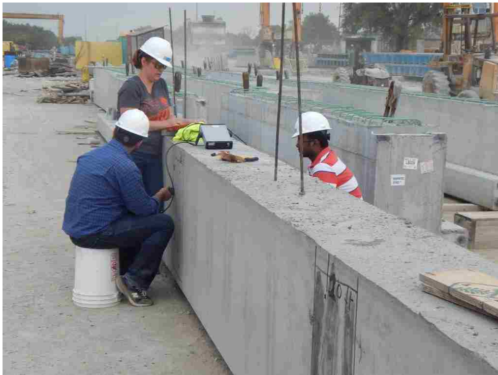
Figure 5.21 On-site UPV testing on beam.
