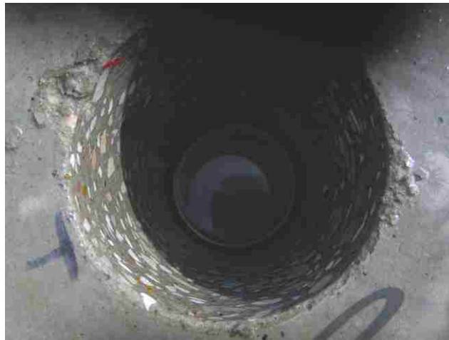
Figure 5.17 Drilled core in beam.
