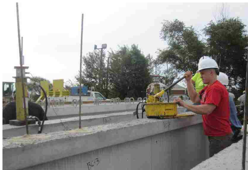
Figure 5.25 Strands being tested using pull-out test.
