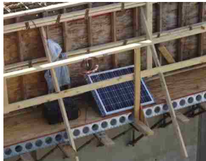
(a) Bent construction (thermocouples)
