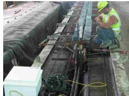
(b) Girders fabrication (VWSGs)
