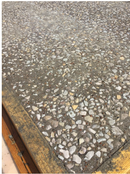
Figure 6-2 Substrate surface preparation
