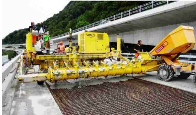
Figure 2-16 Implementation details of UHPC overlay application
