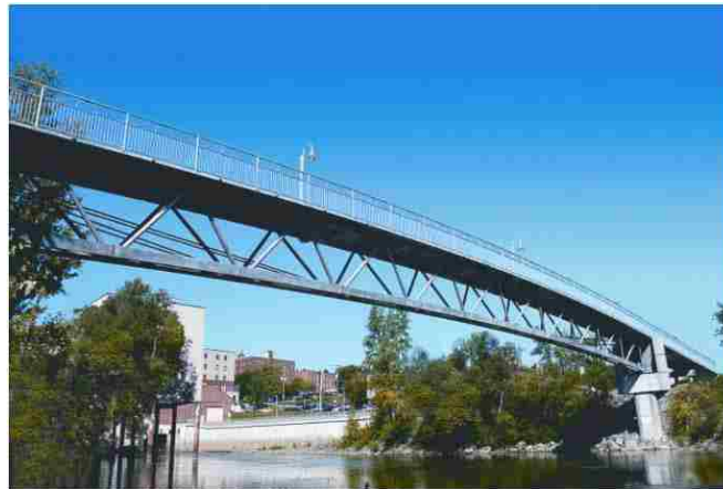
Figure 2-12 Sherbrooke Pedestrian Bridge (Russell and Graybeal, 2013).
