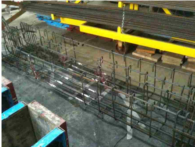
Figure 4.10 Completed Cage for Beam Splice Specimen
