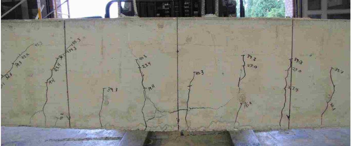
Figure 5.13 Beam Splice Crack Propagation at Failure (RAC50-1)
