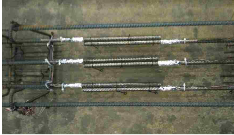
Figure 4.9 Spliced Length with Attached Strain Gauges
