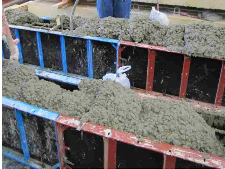
Figure 4.12 Casting of Beam Splice Specimens
