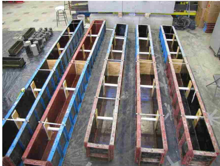
Figure 4.1 Formwork for Casting Pre-Recycled Concrete
