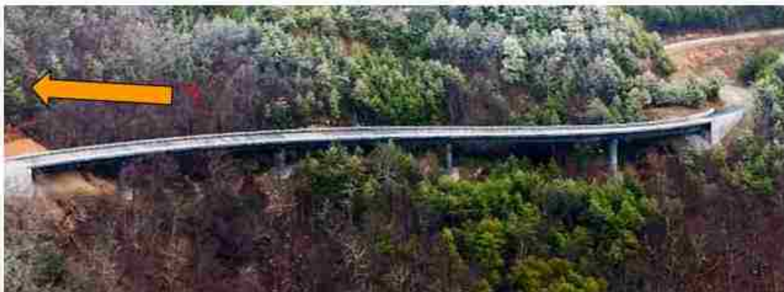
Figure 3.2. Bridge No.2 Side View, Elevation and Surroundings.
