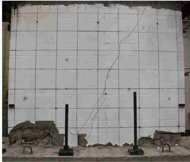
Figure 4.6. Shear Wall One damaged (the shear crack is indicated in green)
