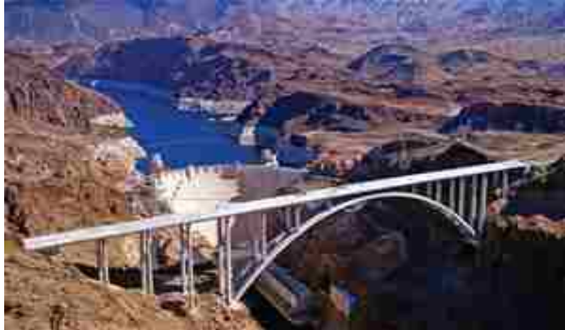
Figure 2.3. Example of Open Spandrel Bridge, Hoover Dam Bypass Bridge, NV
