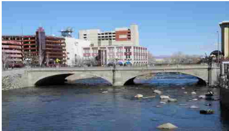
Figure 2.2. Example of a Closed Spandrel Arch Bridge, Virginia Street Bridge, Reno, NV
