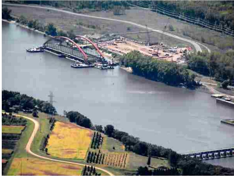
Figure 9.4. Low-Level Transport. Hasting Bridge at the Mississippi River, Furrer and Hasbrouck (2011)
