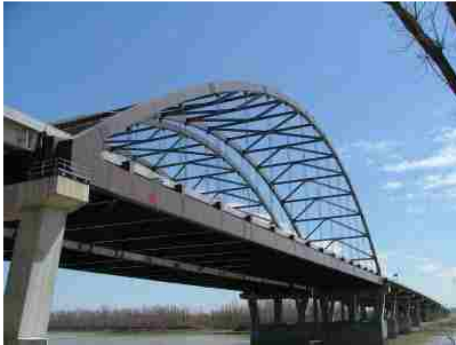
Figure 3.3. Page Avenue Bridge (Rte 364), St. Louis, MO. Photo from: http://bridgehunter.com/mo/st-louis/page/
