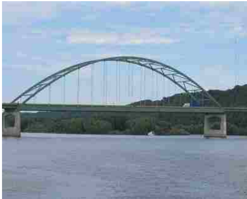
Figure 3.2. City Island Bridge, Dubuque, Iowa. Photo from: http://bridgehunter.com/ia/dubuque/604440/
