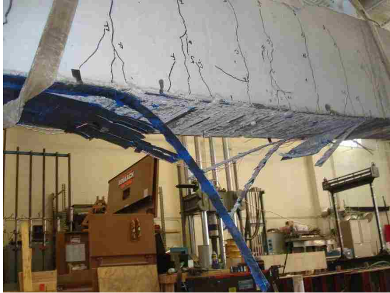
Figure 4.41. Failure of Beam 4
