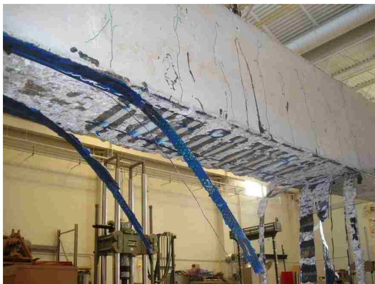
Figure 4.73. Failure of Beam 11
