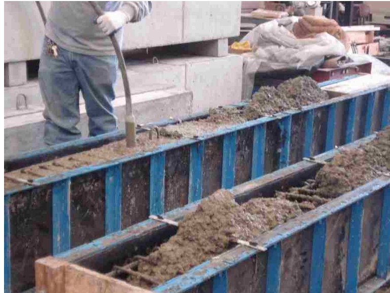
Figure 4.5. Internal Vibration
