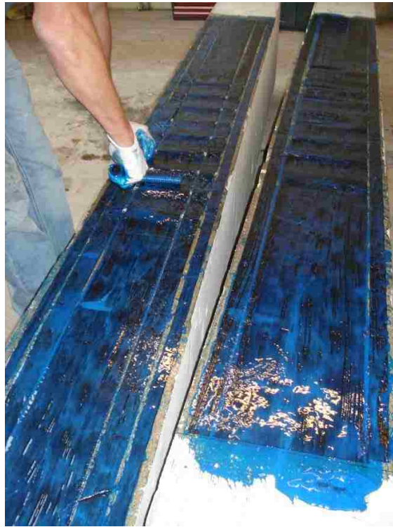
Figure 4.29. Ensuring Proper Bonding
