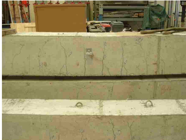
Figure 4.10. Failure of Beam 1
