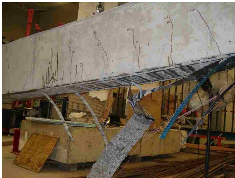
Figure 4.46. Failure of Beam 5
