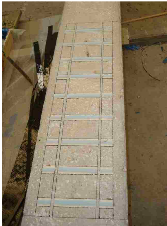
Figure 4.28. Layout of Foam Prior to FRP Application
