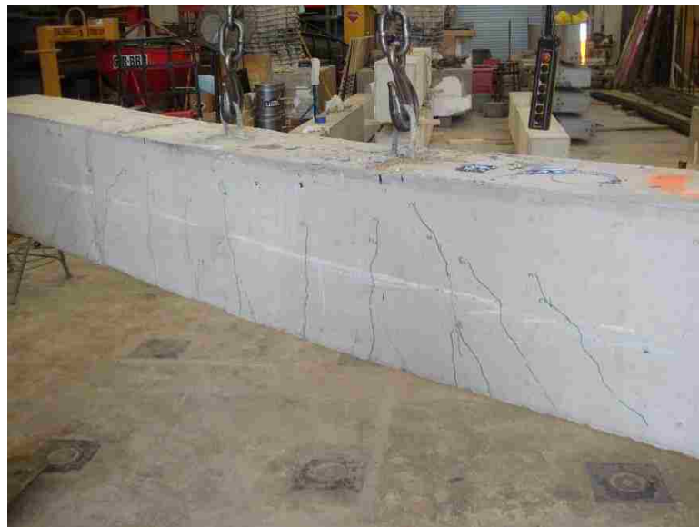
Figure 4.34. Failure of Beam 2
