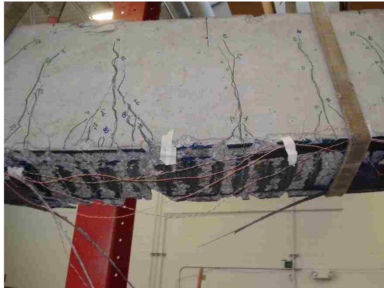
Figure 4.13. Failure of Beam 2
