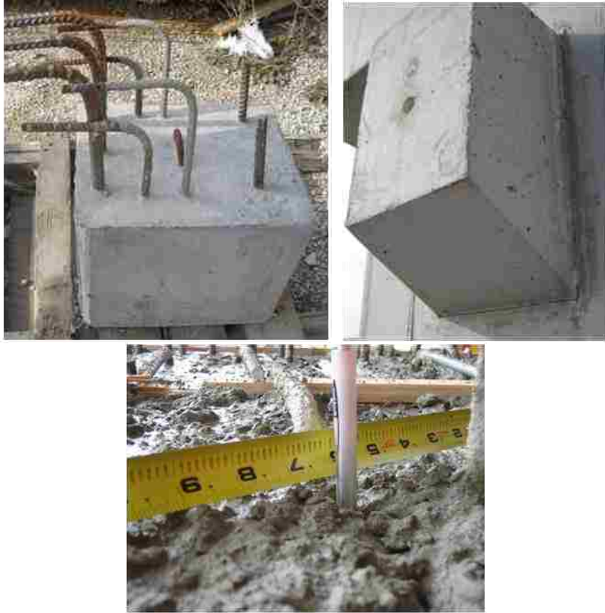
Figure 2.10. Precast facility #1 button corbel (top-left), final placement of corbel (top-right) and precast facility #2 button corbel (bottom)
