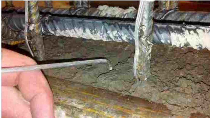
Figure 3.9. Specialized roughening instrument and technique
