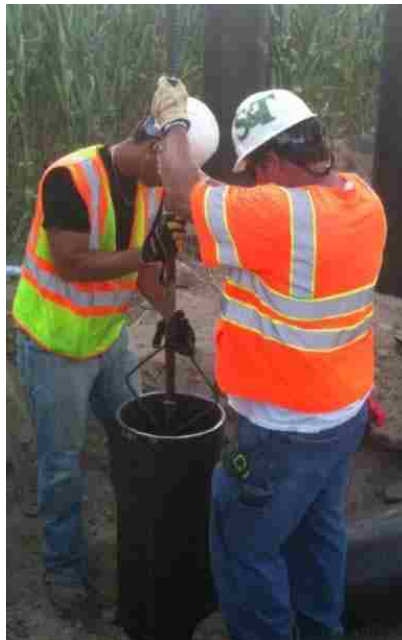
Figure 5.7 Installation of the Center Bar and VWGSs
