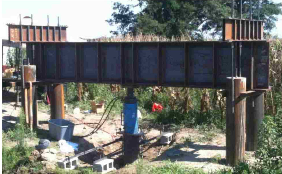
Figure 5.9 Completed A7956 Pile Load Test Set-up
