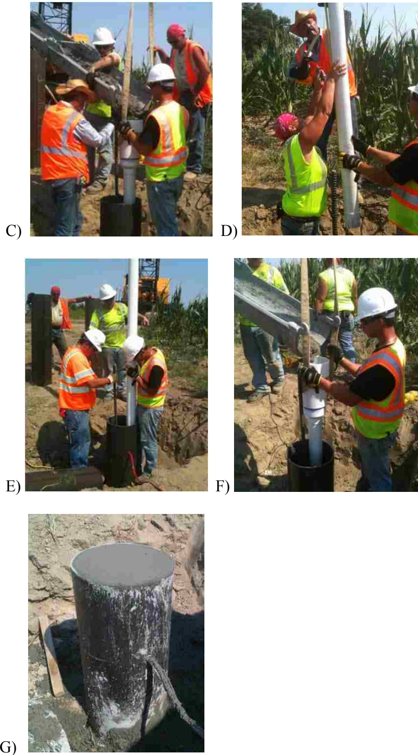
Figure 5.8 (cont.) Process of Test Pile Concrete Placement. (C) Begin Concrete Placement. (D) PVC Tremme Removed and Shortened with Sawzall. (E) PVC Tremme Re-lowered into Test Pile. (F) Resume Concrete Placement. (G) Concrete Placement Finished.
