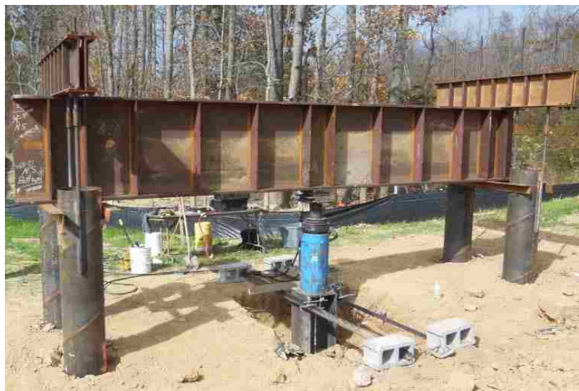
Figure 5.23 Completed A7669 Pile Load Test Set-up
