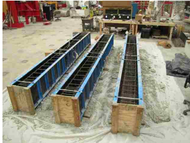
Figure 5.4 – Cages in the formwork
