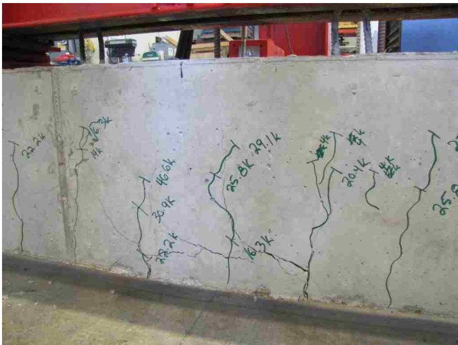
Figure 5.13 – Failed fly ash specimen with no confinement
