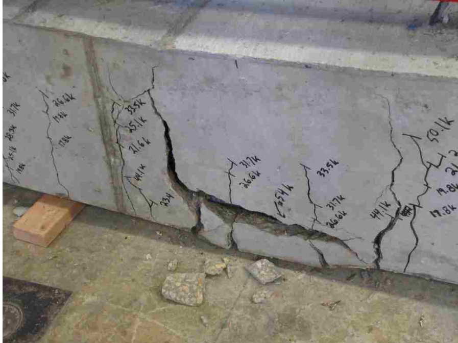
Figure 5.11 – Failed control specimen with no confinement
