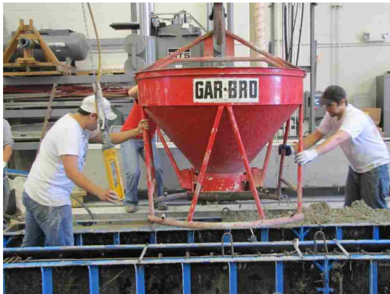
Figure 5.6 – Transferring concrete from the truck to the forms using a bucket
