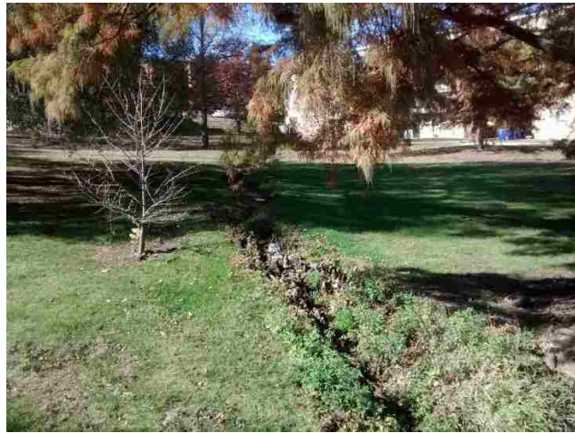
Figure D3. Detention area at the proposed bioretention facility location at the campus outfall in Catchment B.
