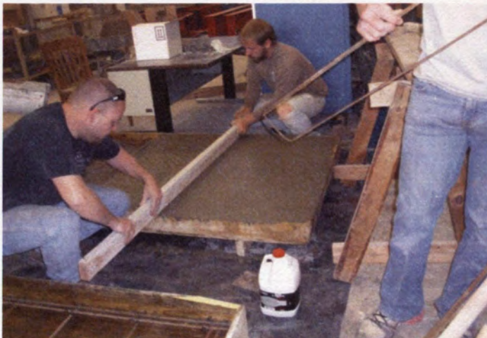
(c) Leveling with Screed
