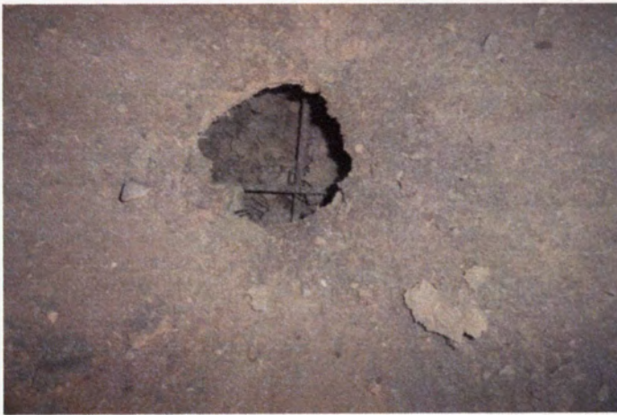
(c) Hole in the Compression Face
