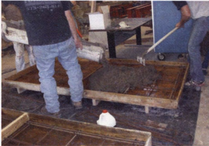
(a) Pouring of SFRC
