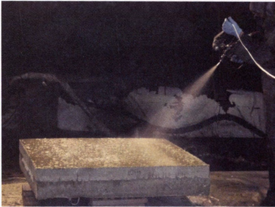
Figure 3.8 – E-Glass DFRP B Application
