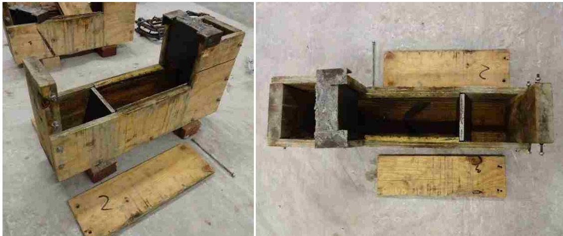
Figure 3.13. Formwork partially assembled for first half of cold-joint specimen
