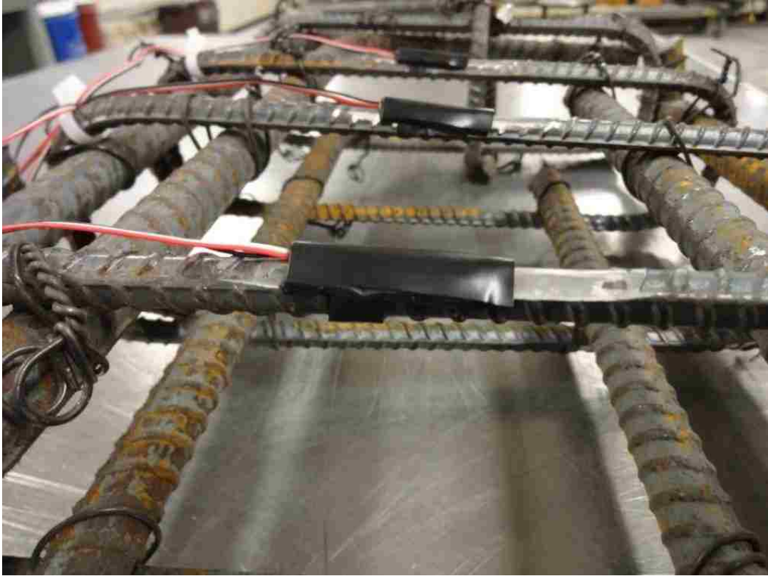
Figure 3.21. Strain gages and protective coating applied to reinforcement
