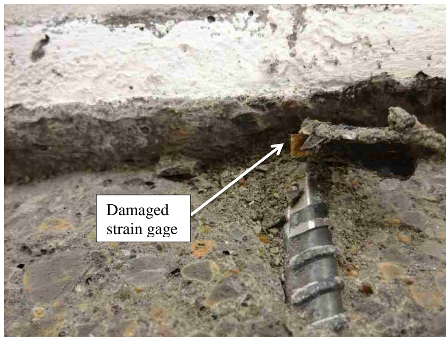
Figure 3.24. Typical damage to strain gage at conclusion of testing
