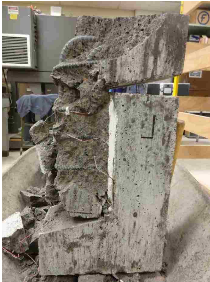
Figure 3.40. Specimen S-CL-CJ-R-17-2 with spalled concrete removed and no shear failure visible
