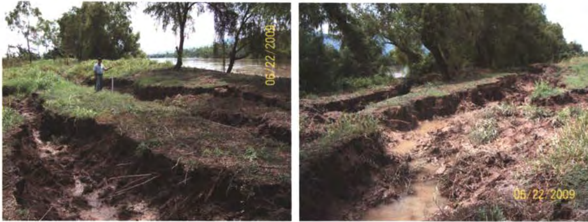
Figure 5-6: Lateral Spreading along the Ulua River
