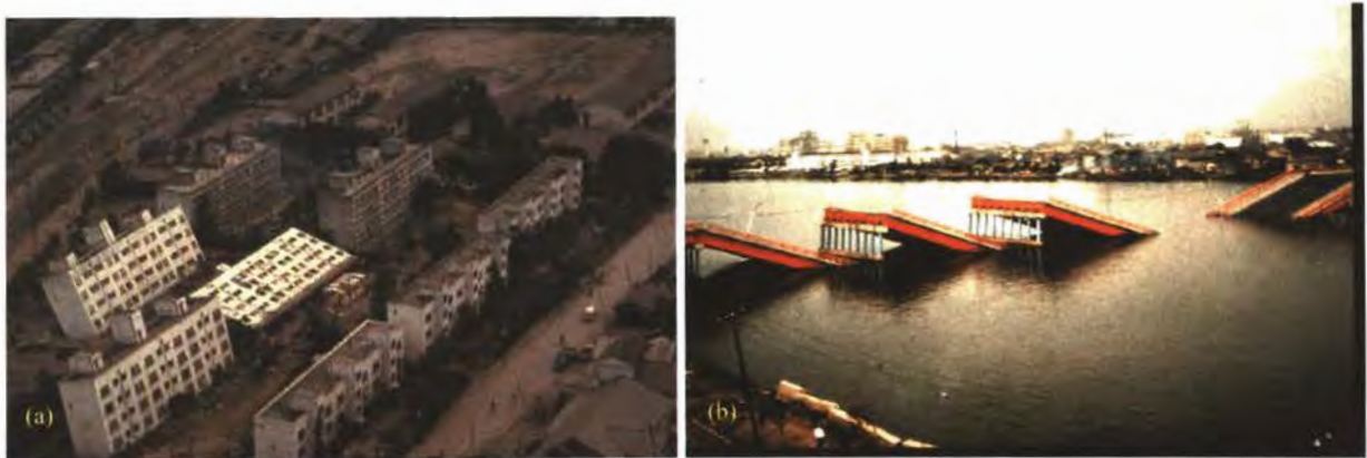
Figure 1-2a,b: Typical damage from 1964 Niigata, Japan Earthquake (a) factory (b) Shinano River Bridge ( http://www.johnmartin.com/earthquakes/eqshow/images )
