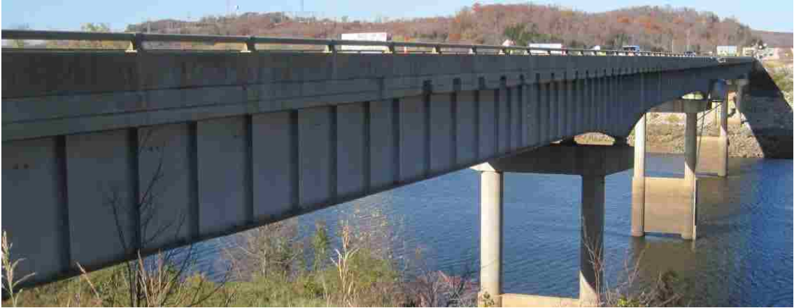
Figure 3.14. Bridge A1479 Side View
