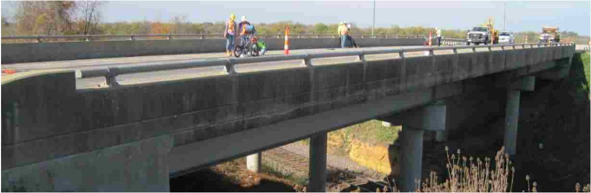
Figure 3.33. Bridge A1297 Side View
