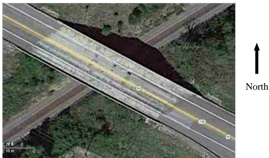
Figure 3.34. Bridge A1297 from Satellite Imagery [51]
