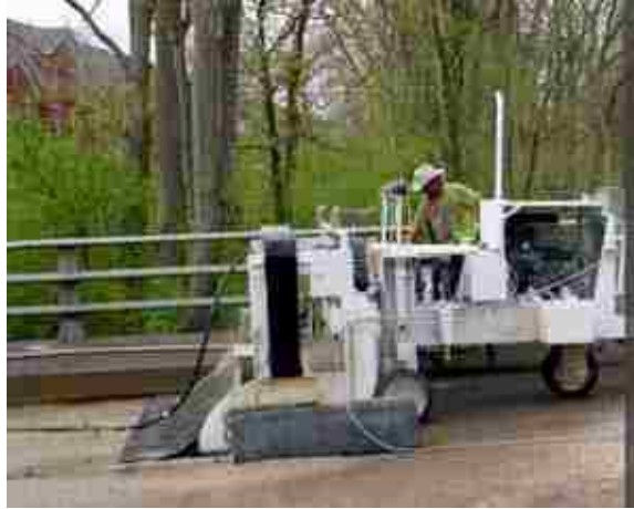
Figure 2.12. Hydrodemolition Machine [45]
