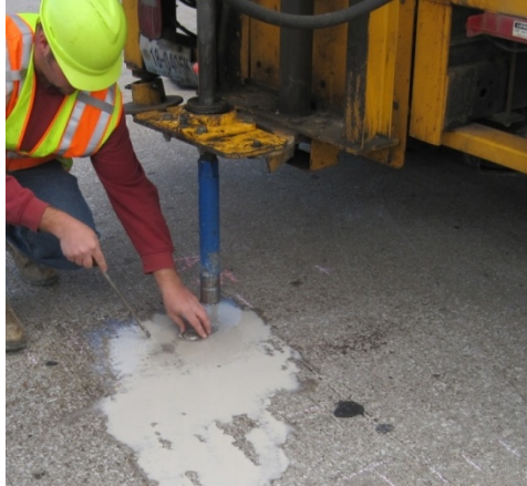
Figure 3.6. Extraction of Cores
