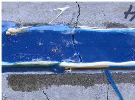
Figure 5.14. Crack pattern difference between Beam # 4 and Sensor # 3
