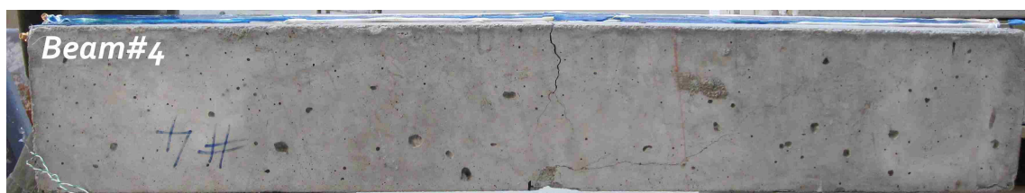
Figure A.3. Beam#4_ PC- Primer Pretreated _ Structural Epoxy
