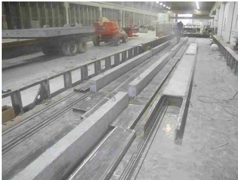
Figure 4.9 – Beams After Form Removal and Before Instrumentation
