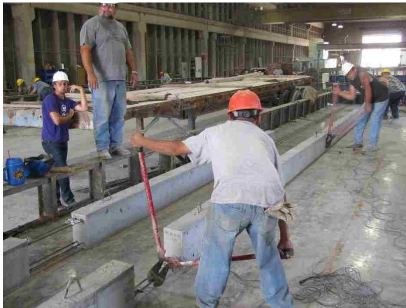
Figure 4.10 – Bolt Cutting Strands at Release
