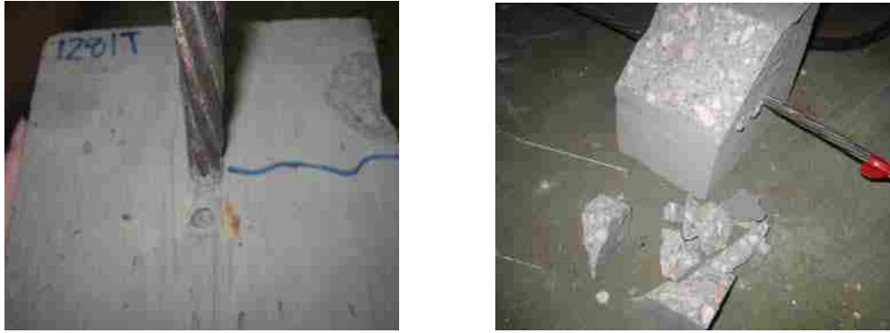
Figure 4.17 Examples of spalling noted after heating process (left: local spalling, right: serious sloughing/explosive spalling)
