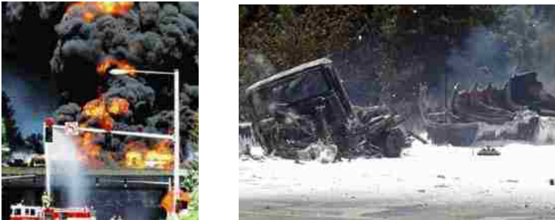
Figure 6.14 Bridge fire caused by a tractor trailer carrying gasoline which occurred on U.S. Interstate-5 near Lynnwood, Washington (Washington State Department of Transportation, 2003)
