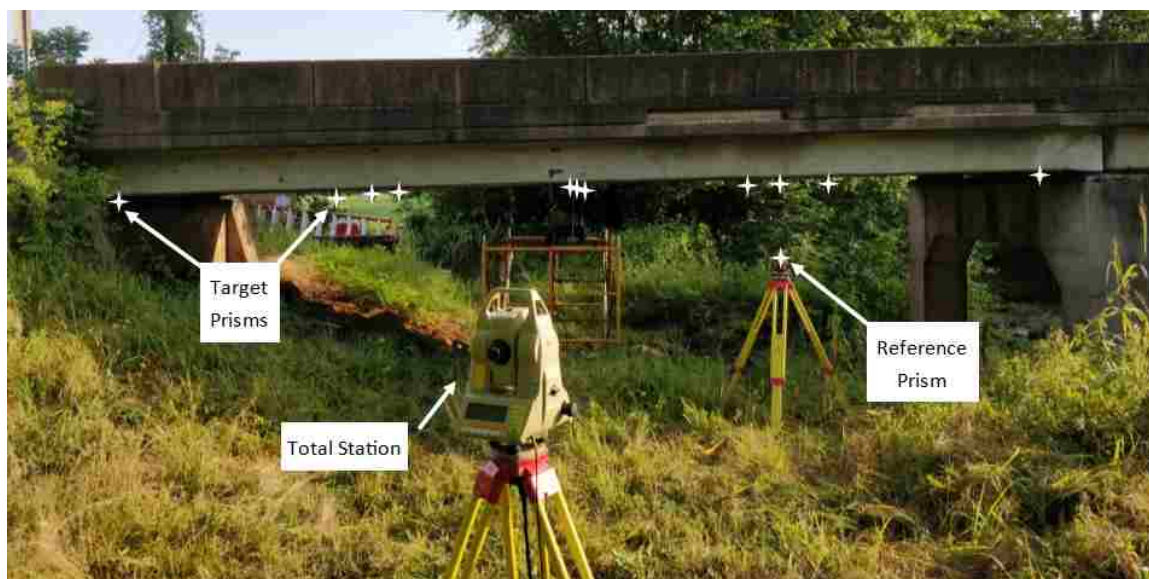
Figure 5.4. Total Station Setup
