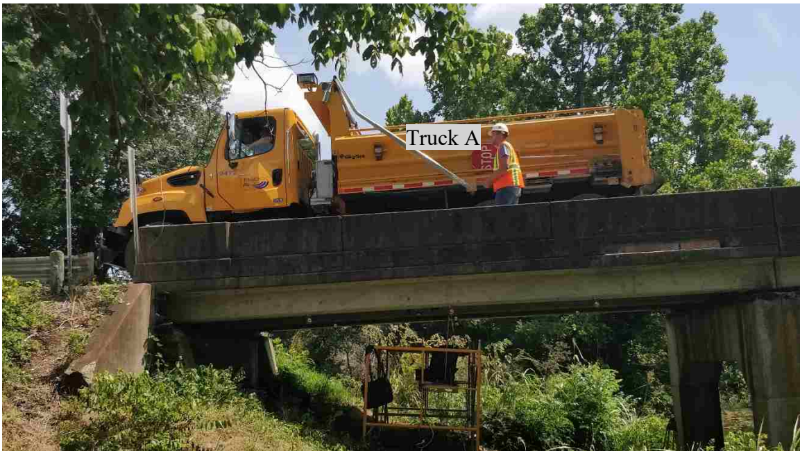
Figure 5.8. Truck on Span 4 for Load Test
