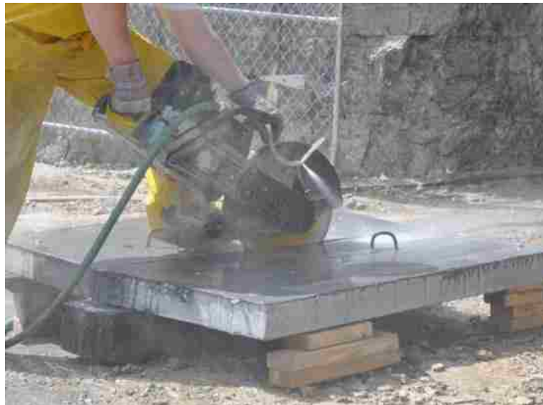
Figure 5.22. Half panel fabrication process
