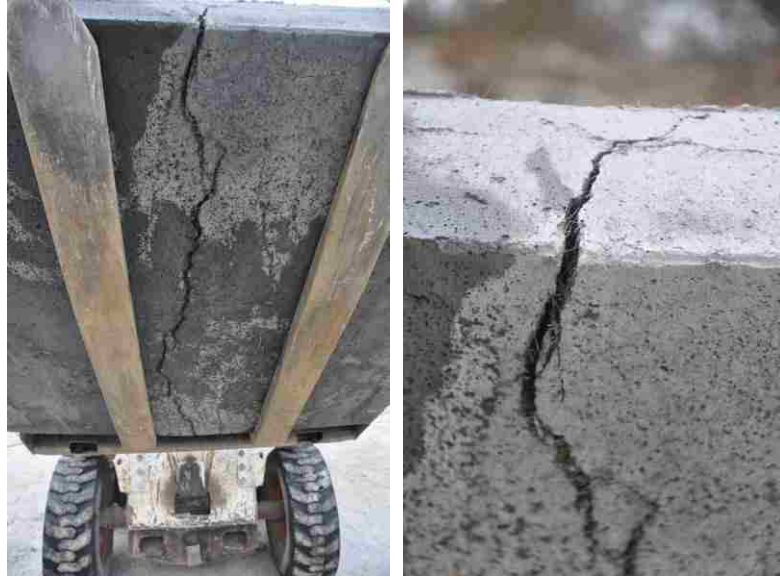
Figure 6.28. Cracking on the tension face after testing
