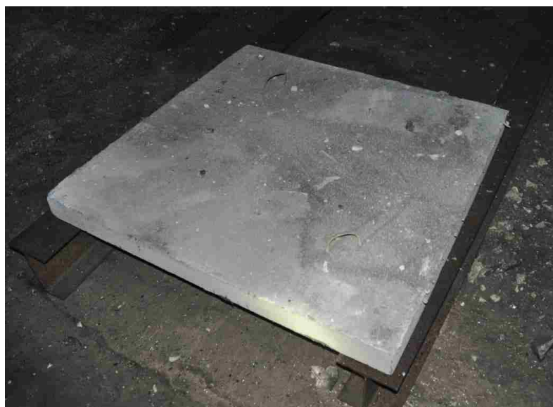
Figure 6.24. Top face of B-1-6F-3.5 after first detonation
