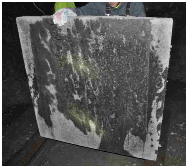
Figure 6.25. Bottom face of B-1-6F-3.5 after first detonation
