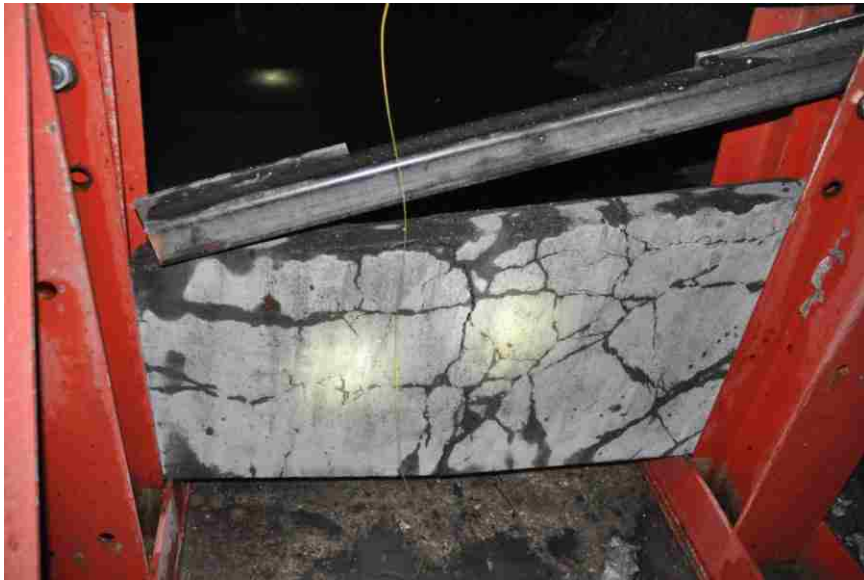
Figure 6.45. Back face of H-1-2F-3.5 after detonation
