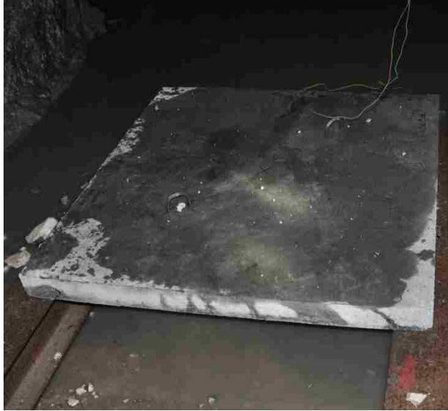
Figure 6.18. Top face of B-3-2F-3.5 after detonation
