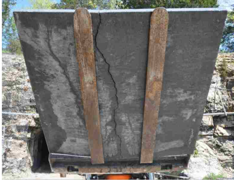
Figure 6.35. Tension face cracking of B-6-6F-2 after detonation
