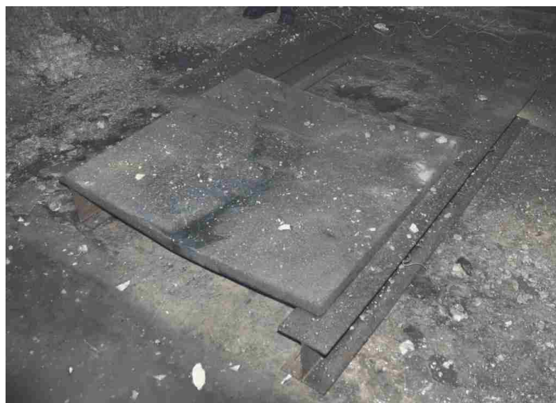
Figure 6.32. Top face of B-6-6F-2 after detonation
