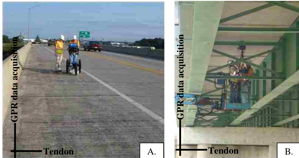
Figure 3.7: Process of acquiring GPR data in the longitudinal direction (A. Top surface acquisition using a cart, B. Bottom surface acquisition using a survey wheel apparatus)
