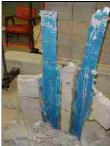
(a) Surface Laminate Retrofit
