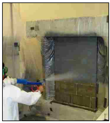
(b) Application of Polyurea
