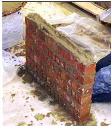
(c) Bed-Joint Construction
