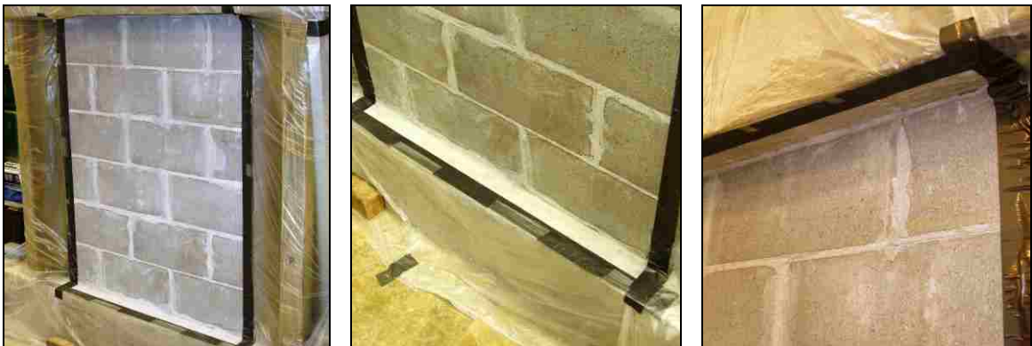
(a) Face of URM Wall
