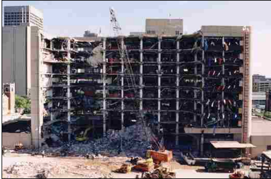
Figure 1.1. Damage to Alfred P. Murrah Building (FEMA, 2003)
