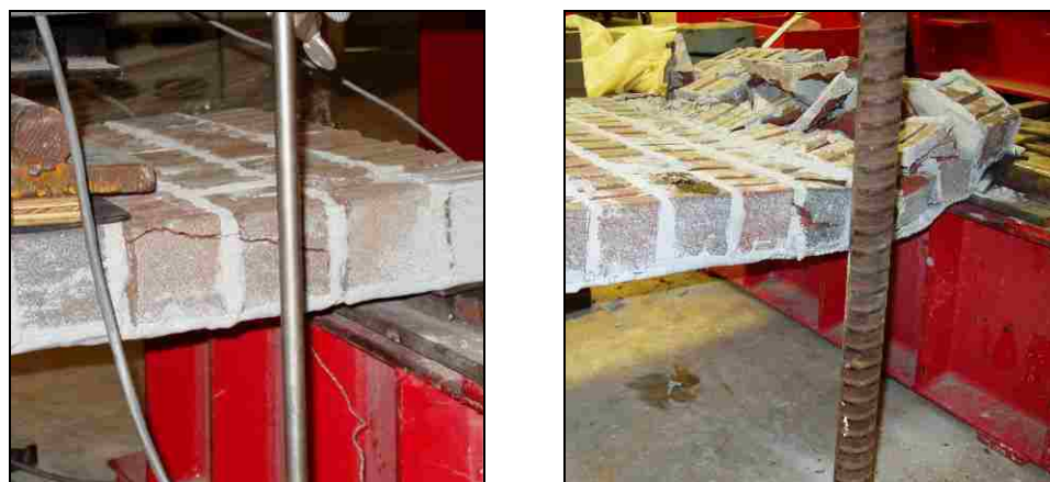
(a) Flexural-Shear Cracking
