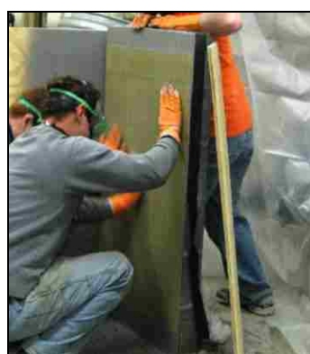
(b) Embedding FRP Grid
