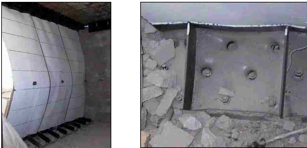
Figure 2.3. Steel Plate Catcher System (Bogosian and Crawford, 2000)
