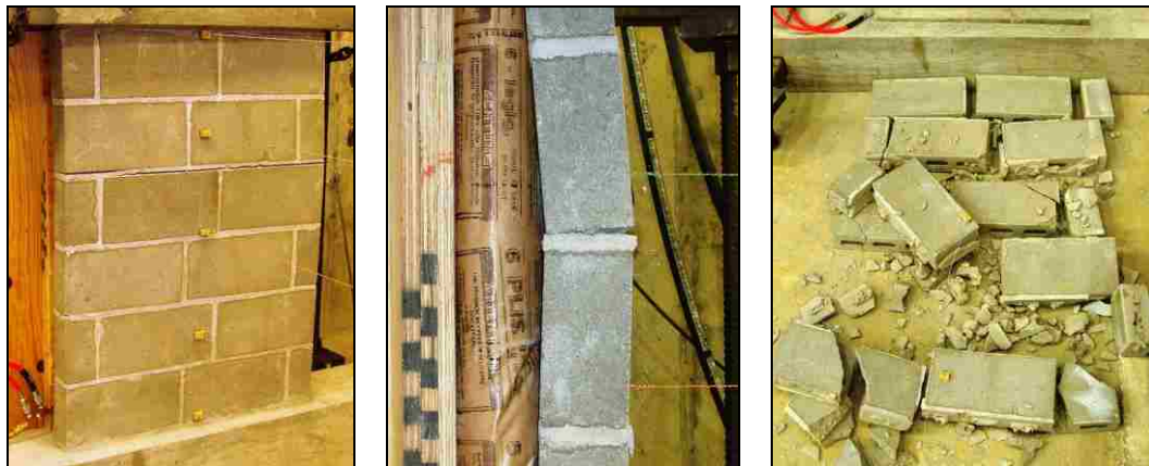
(a) Horizontal Cracking (b) Rigid-Body Behavior (c) Debris Scatter
