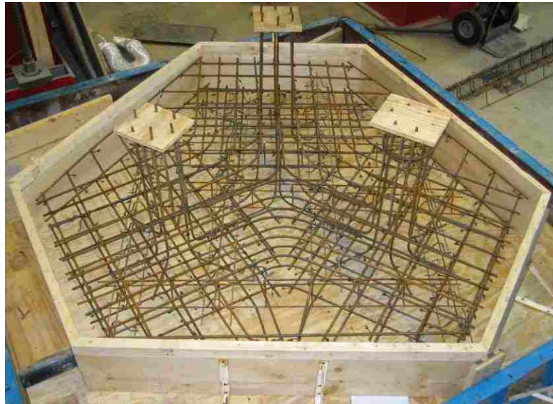
Figure 5.2. Formwork and Reinforcement for Footing
