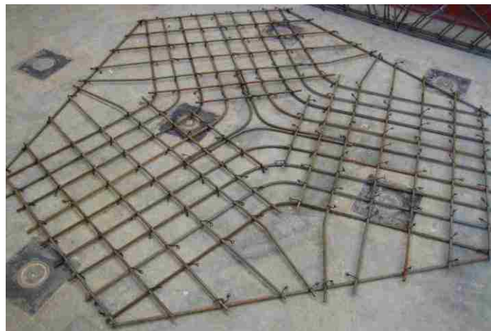
Figure 5.1. One Layer of Reinforcement for Footing and Slab
