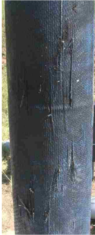
Figure 6.5. Damage to Front of Column 3 after 1 st 4 lbs Blast
