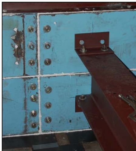
Figure 3.8. Purlin Support Beam to Chamber Connection
