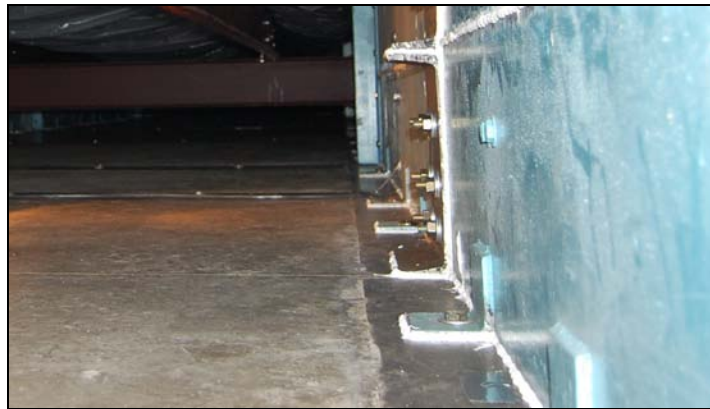
Figure 3.7. Chamber-to-Floor Connection
