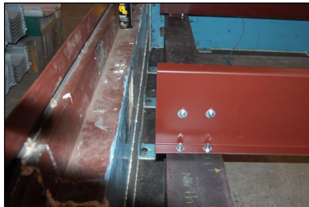
Figure 3.1. Flange-Bolted Connection
