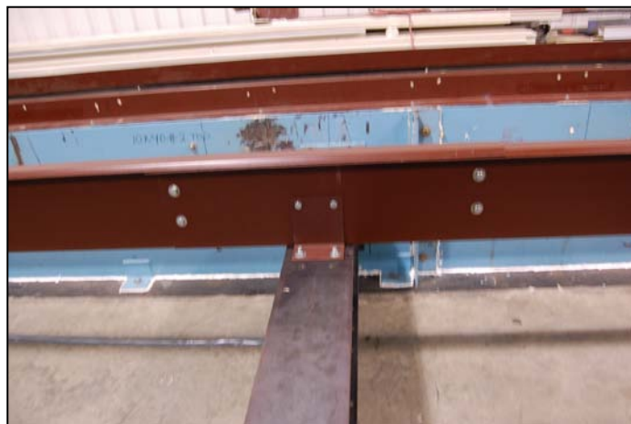
Figure 3.10. Continuous Span Typical Lap Connection
