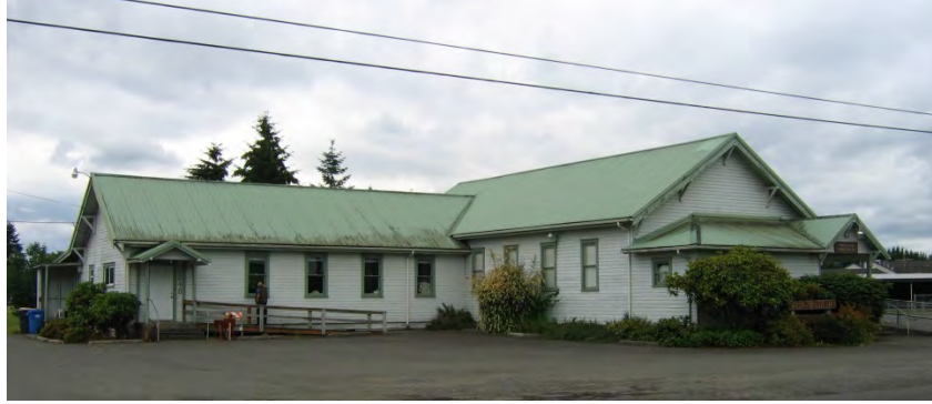
Figure 5.9: Ford's Prairie #33 in Lewis County (Example of a hall with a commonly observed L-shaped extension off of the main elongated rectangle)
