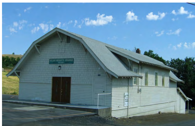
Figure 5.16: Selah Heights #608 in Yakima County (Example of gambrel roof form)
