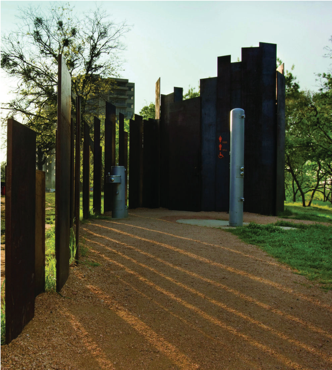
figure 48: Trail restroom on Lady Bird Lake In Austin, Texas
