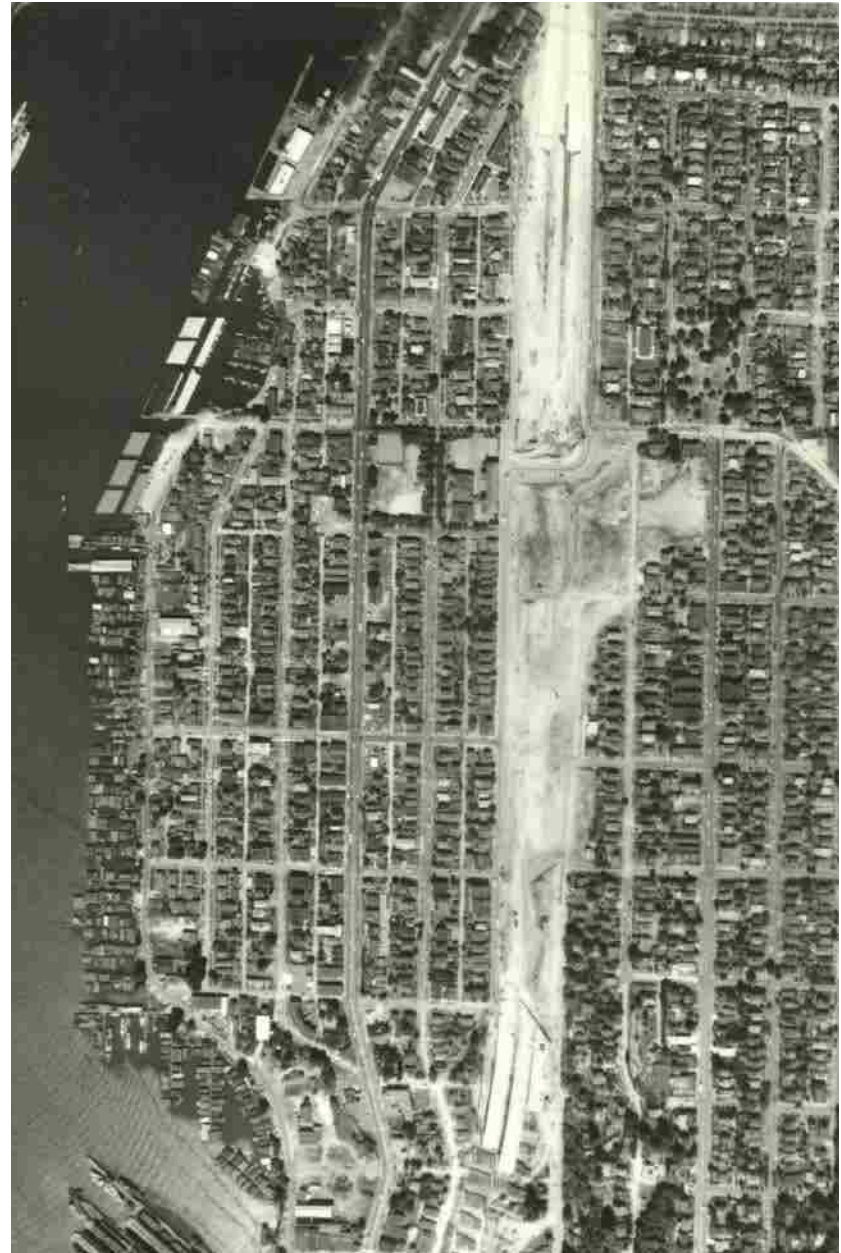
figure 3: 1961 aerial image of I-5 construction in Seattle
