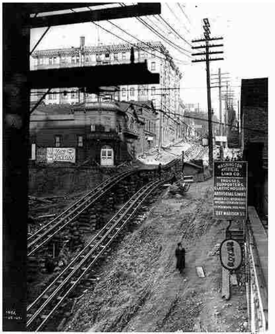
Madison Under Construction
