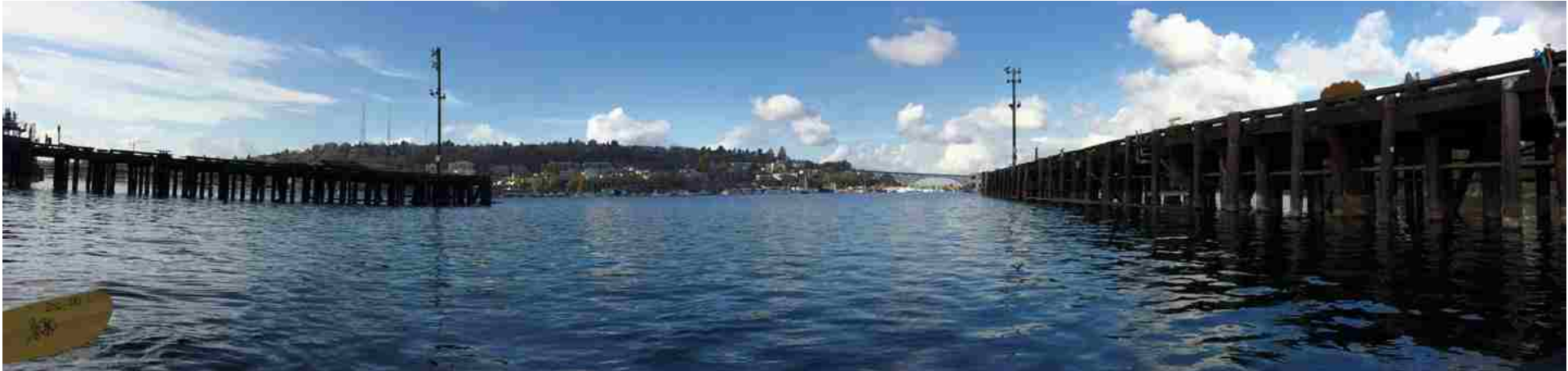
Figure 20. View looking west, between the two piers.
