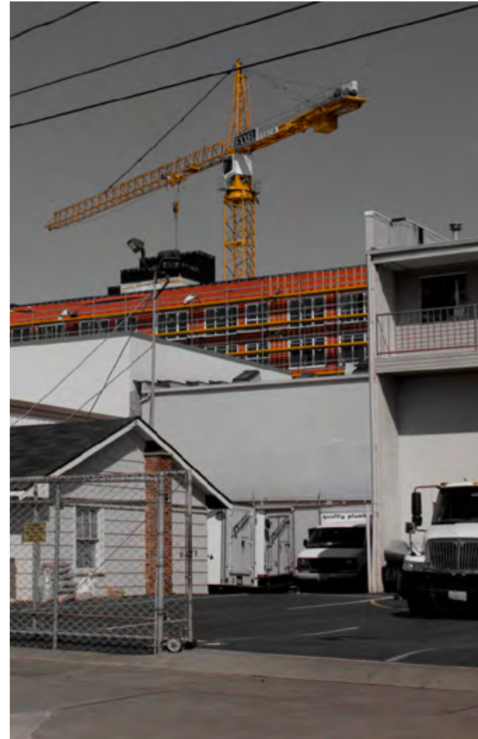
figure 1.03 Construction on the fringe
