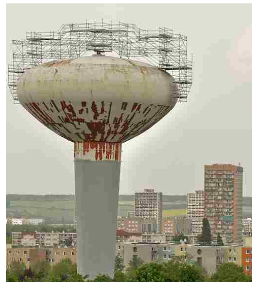
Figure 5.14 Scaffolding conforming to unique form
