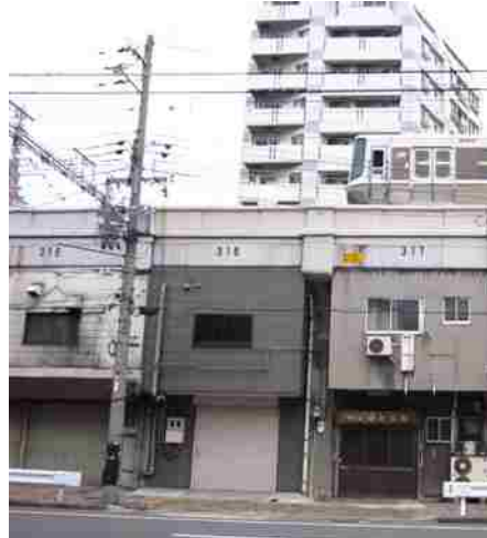
(b) (infra)structural gaps
