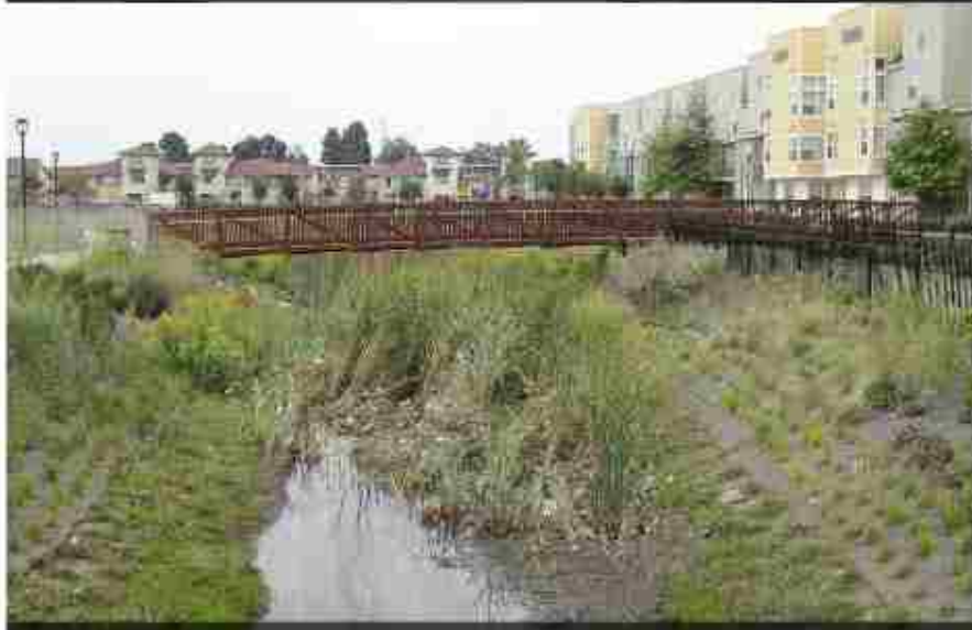
a. Restored, Natural Portion North and West of the Project Site
