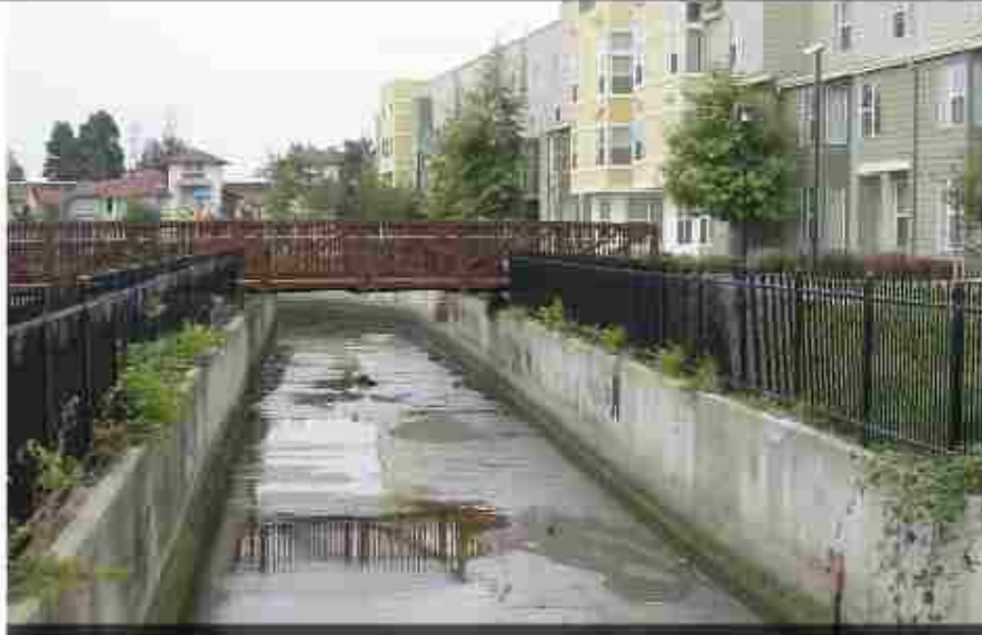
a. Concrete-lined Portion North of the Project Site
