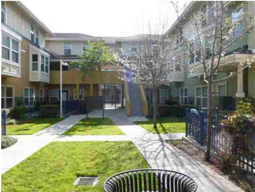
Image 33: Placemaking on the Patio (Lower Right)
