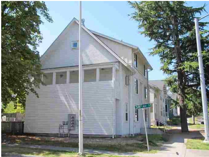
Image 23: Four-plex Buildings Attempting to Hide Stairs by Design
