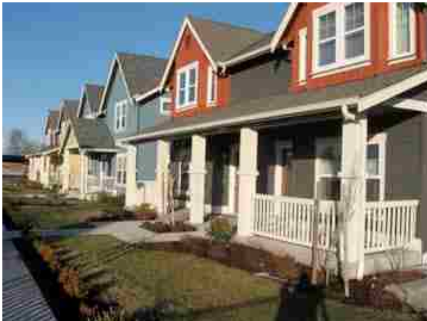
Duplex residences with porches, landscaping and sidewalk that buffer the homes from the street
