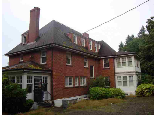
Figure 5 Current conditions of structures on the island including (top left) the Luhr Creek Residence, (top right) the warden's mansion and (below) the community center. Photos by author.
