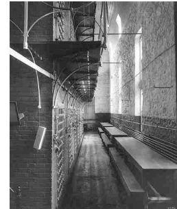
Figure 4 Interior of the original cell house completed in 1875. The structure was demolished in 1937. Image courtesy of MOHAI.
