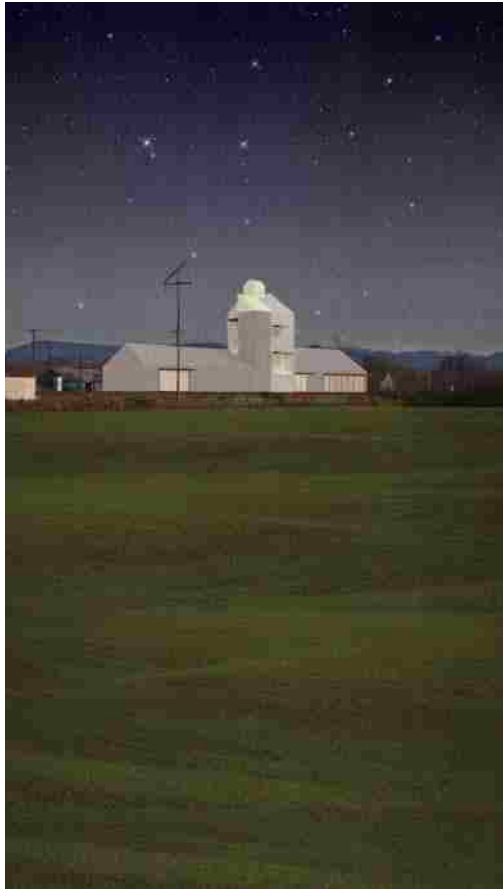
56. View of proposed facility at night from across the fields
