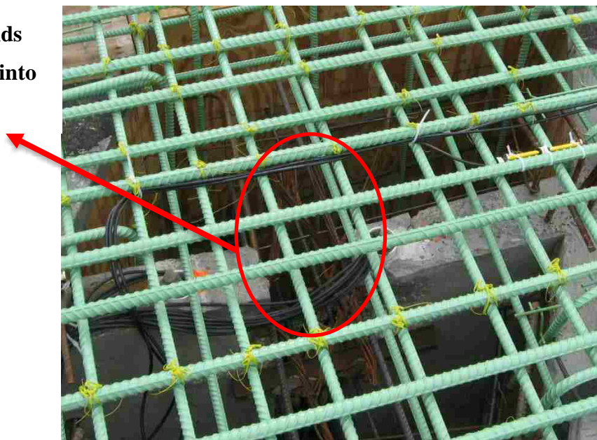
Figure 2.14 Intermediate bent in highway-50 Bridge with top strands highlighted
