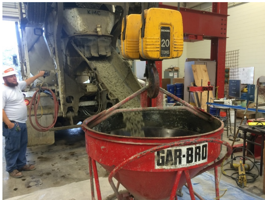
Figure 5.1 Concrete being delivered by a ready mix truck
