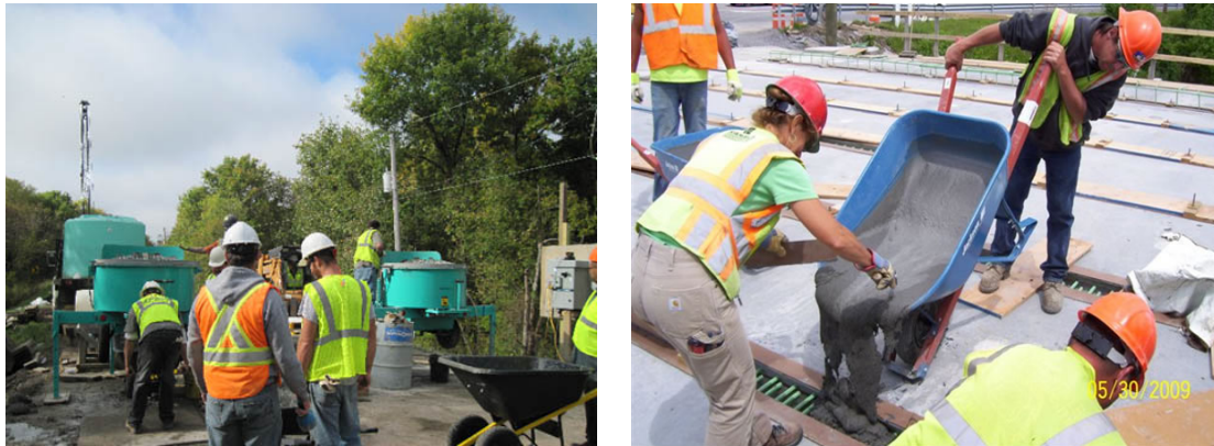
Figure 2.2 Batching and casting UHPC at site (FHWA, 2016)
