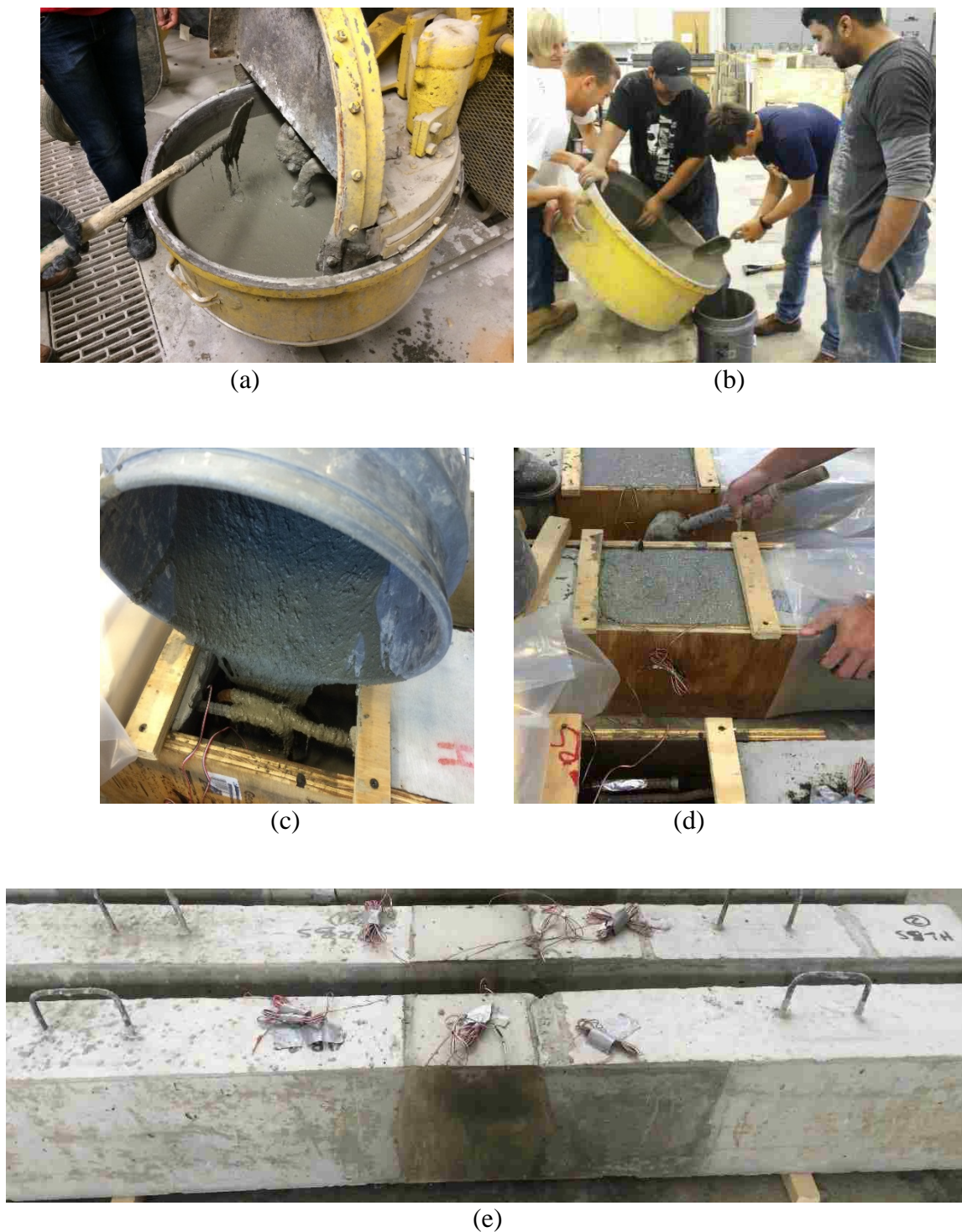
Figure 5.6 Various stages of UHPC batching and casting
