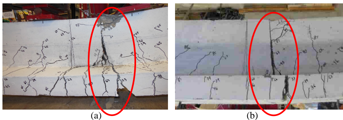
Figure 6.24 Failure mode (a) B-4-U-MB-M (b) B-5-U-U-M
