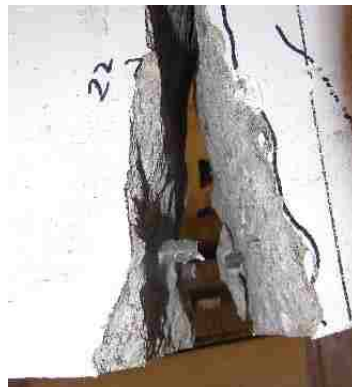
(d) Specimen B-21-U-S-H showing rebar rupture Figure 6.18 UHPC hairpin specimens at failure
