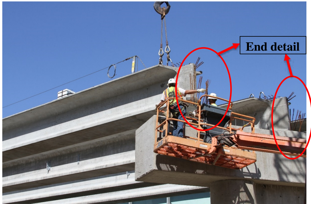
Figure 2.13 Girder erected in position for Highway 50 Bridge with MoDOT end girder detail
