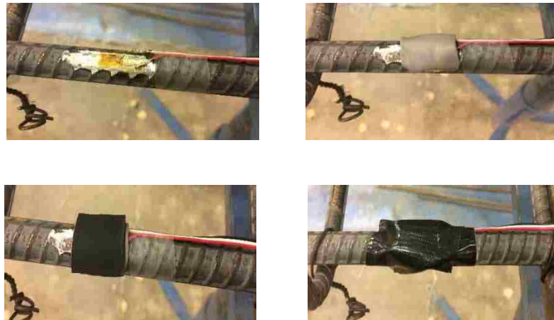
Figure 5.10 Strain gauge installation
