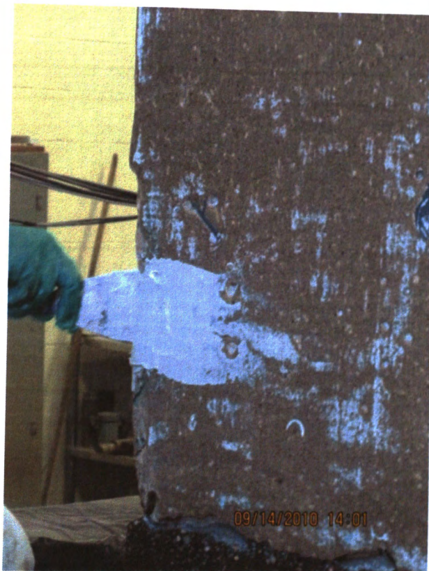
Figure 4.20. Application of MBrace ® Putty
