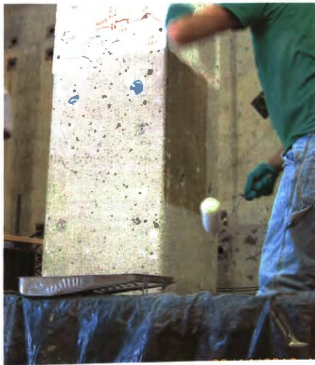
Figure 4.19. Application of MBrace® Primer
