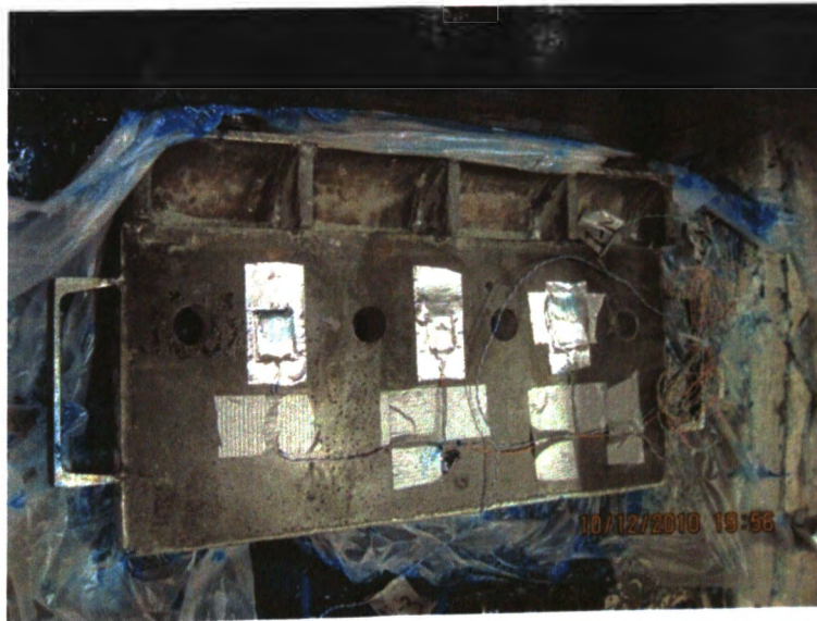
Figure 4.22. Temporary Placement of Anchorage Over “Wet” Saturant
