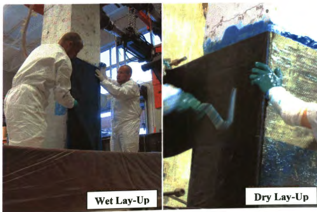
Figure 4.21. Installation of CF 130 Carbon Fiber Sheets
