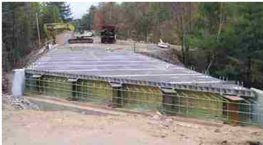
Figure 2.8: DuraSpan® FRP Bridge Deck Panels (Bank, 2006)
