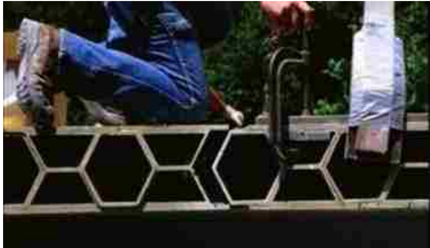
Figure 2.6: Superdeck Panels used in the West Virginia Bridges (Hastak et al., 2004)
