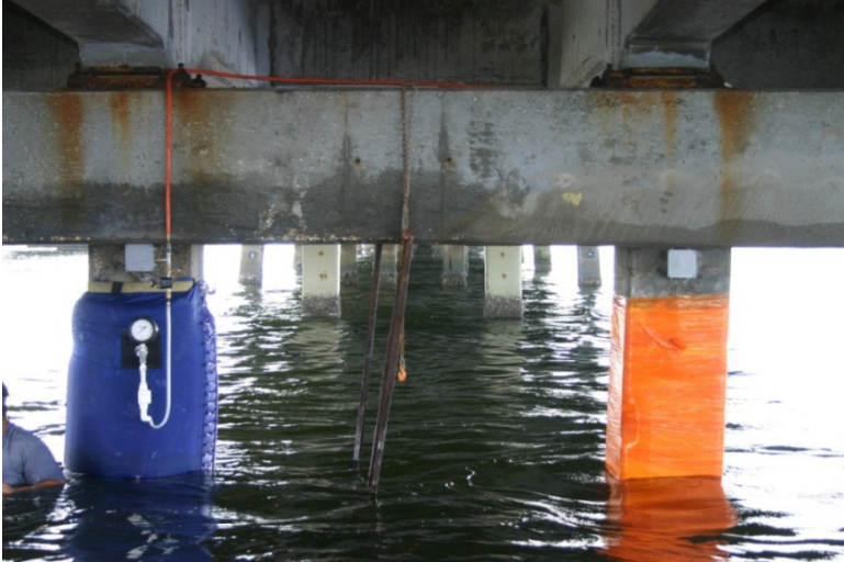
Figure 5.14 Pressure bag applied to the wet layup pile at 14.5 kPa.
