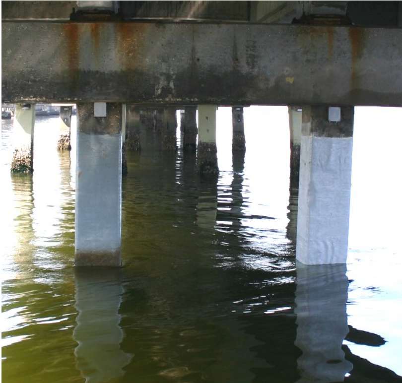
Figure 5.15 Piles after FRP repair with UV coating.
