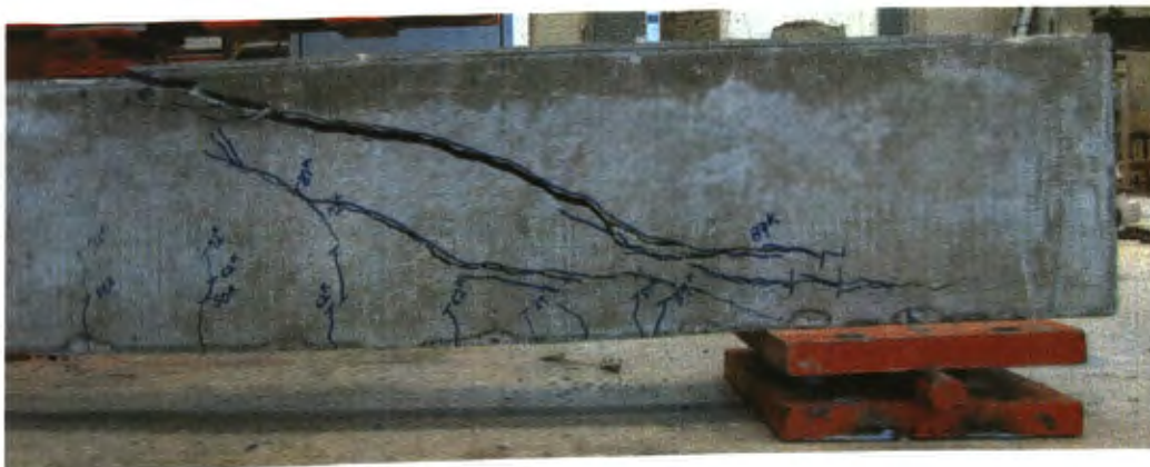
Figure 6.45. Control-NS-3 Beam at Failure
