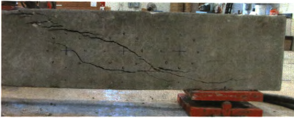
Figure 6.43. Control-NS-1 Beam at Failure
