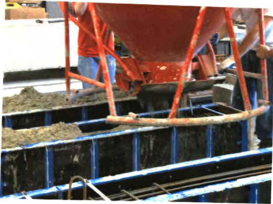
Figure 6.11. Placing Concrete
