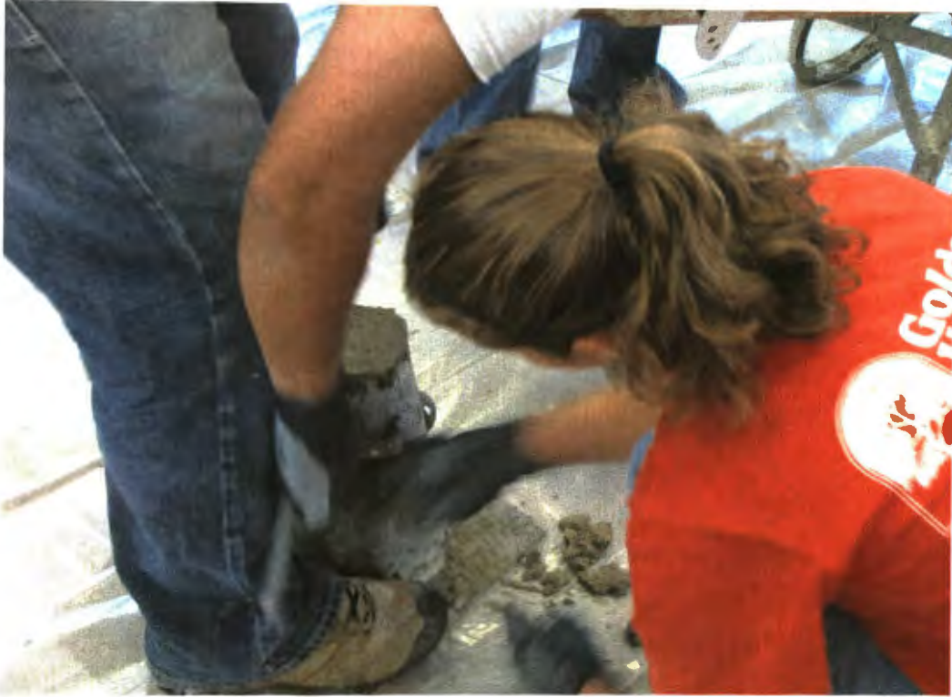
Figure 6.9. Initial Slump Taken
