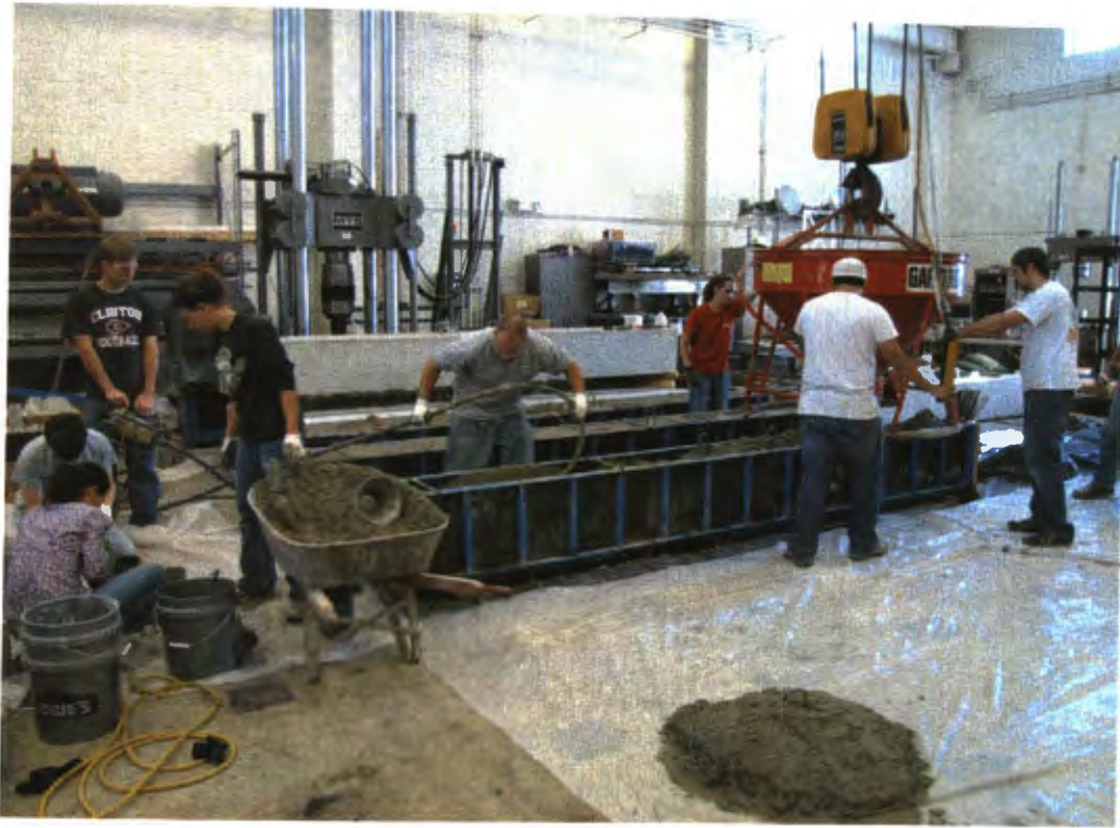
Figure 6.17. Concrete Placement Operations
