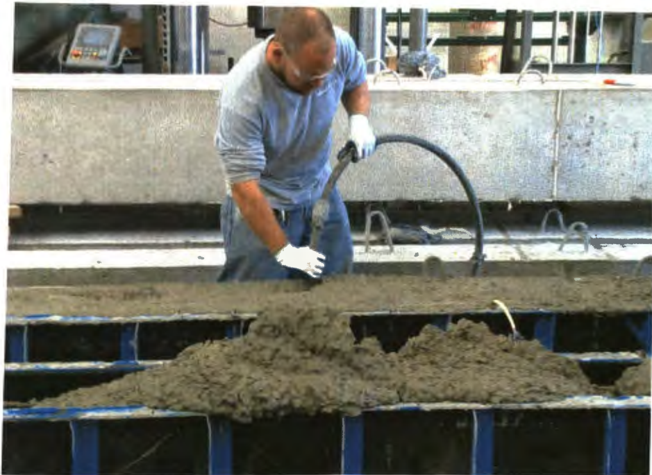
Figure 6.12. Vibrating Concrete
