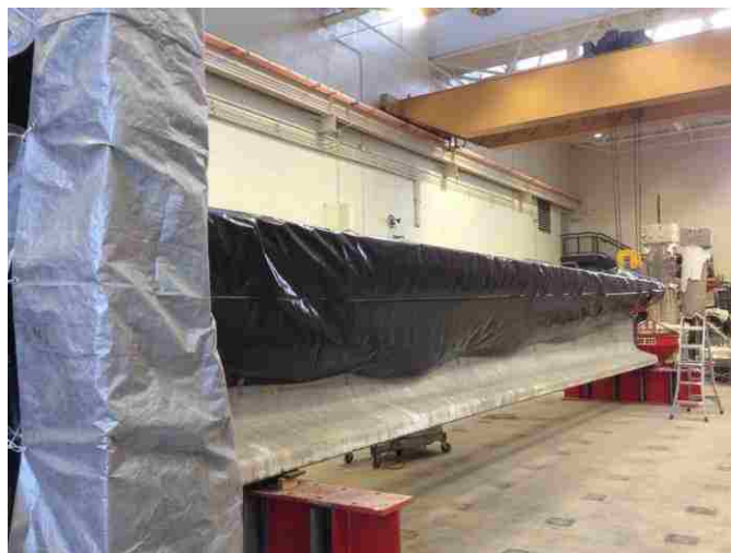
Figure 3.16. Tarping of CIP Deck
