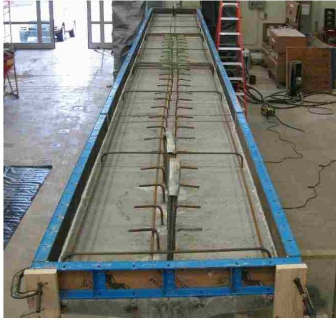
Figure 3.13. CIP Deck Preparation
