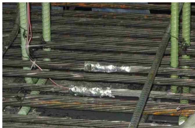
Figure 3.7. Strain Gauge Installation
