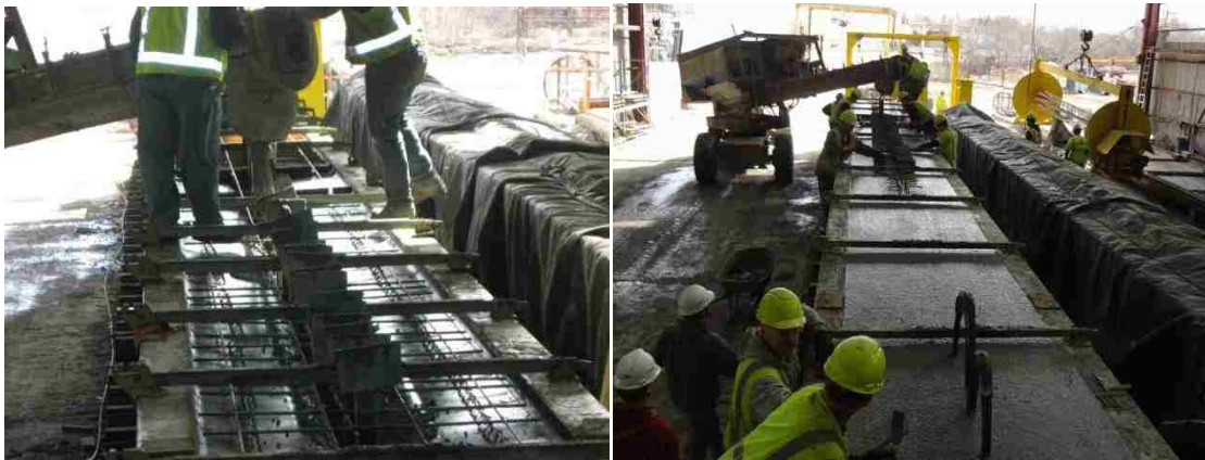
Figure 3.8. Fabrication of Test Girders
