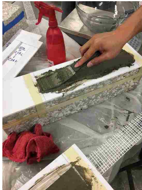
Figure 3.9. Application of first mortar layer to concrete prism
