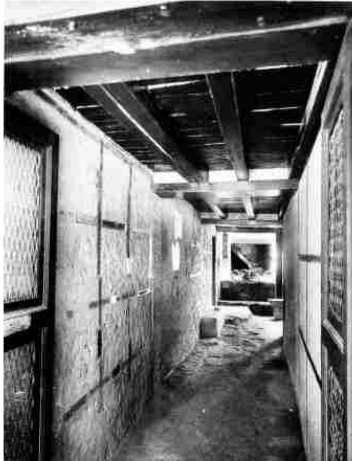
Figure 5.6. An interior hallway in the House of Opus Craticium at Herculaneum (Meiggs 1982:pl.8).
