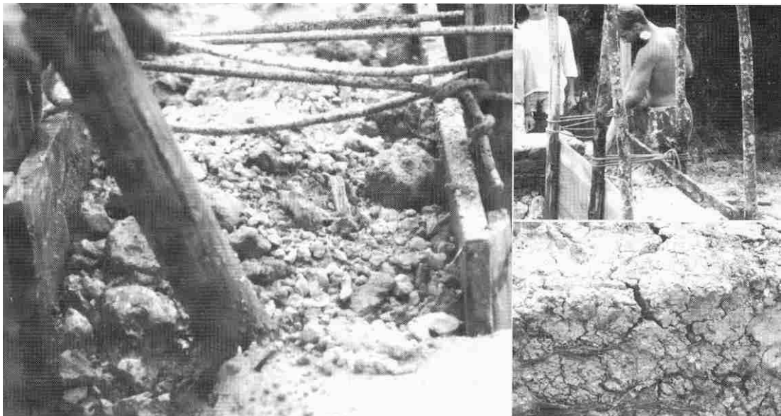
Figure 5.8. The construction of pisé walls at Allumiere using traditional techniques (Genovesi 2001:314).
