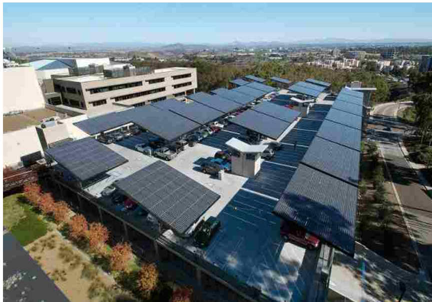
Figure 1.16. An image of the USCD microgrid [47].
