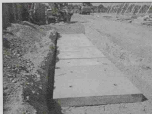
Figure 4.8: The pipes protection
