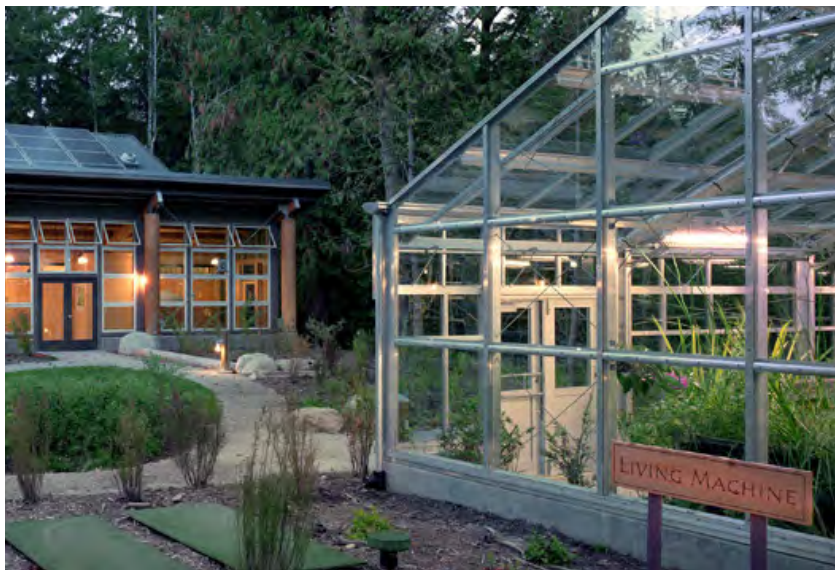
figure 37: living machine - IslandWood | Seattle, Wash
