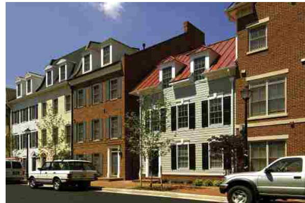
Figure 5.1: Chatham Square street facades
