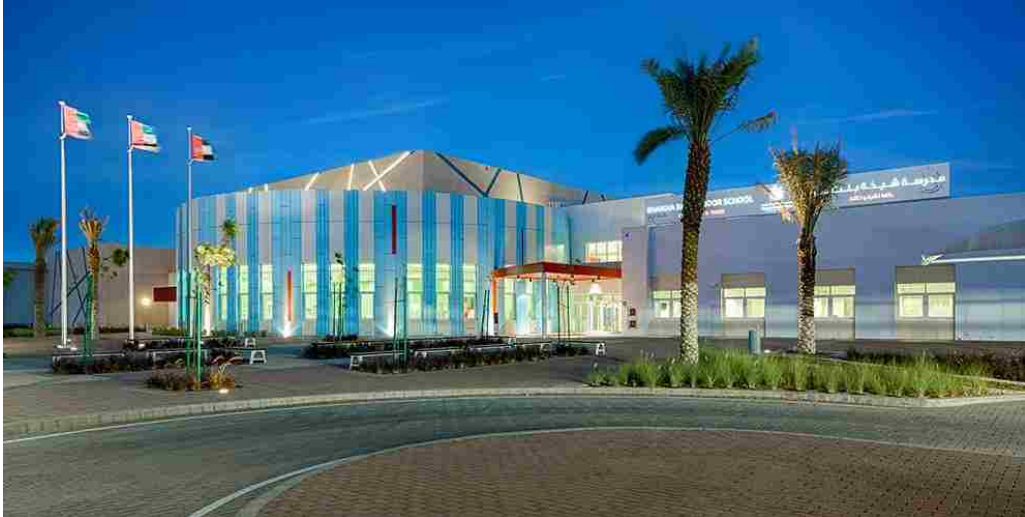
Figure 3.4: Front Entrance of Sheikhha Bint Suroor Public School (KEO, 2017)
