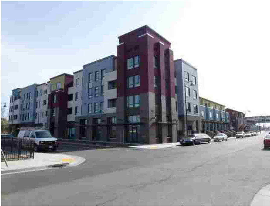
Image 45: Phase VI Building with Saturated Paint Colors
