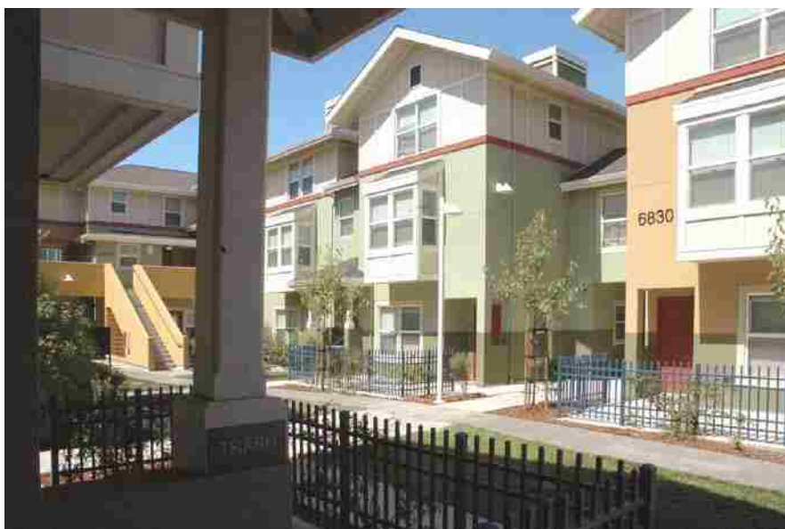
Image 44: View of Court from Corridor Balcony in Elevator-Served Building
