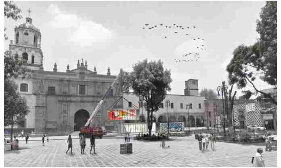
Fig: 8.6 Gallery Constructed on Site
