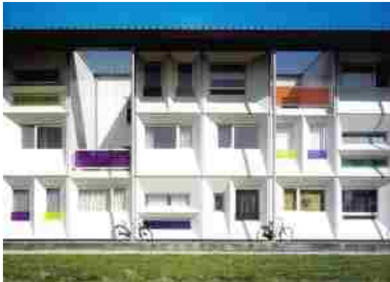
Fig: 4.6 Application of Building Container System
