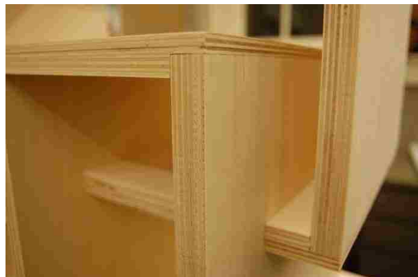
Fig. 9.7 Intersecting and emerging joinery conditions
